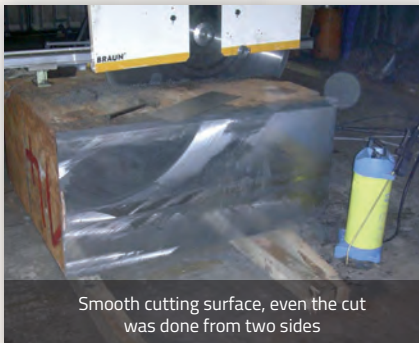
Cutting a vessel of a research reactor from inside (nuclear research institute Riso, Denmark)
