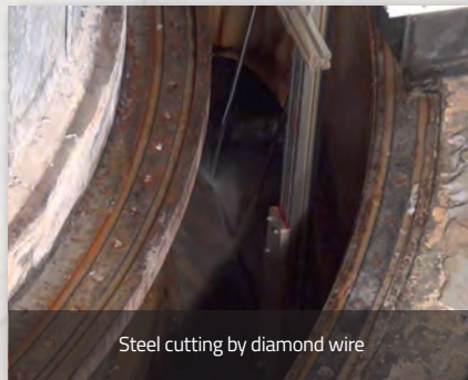
Segmentation of a nuclear submarine by Braun mobile steel cutting saw BKS12
