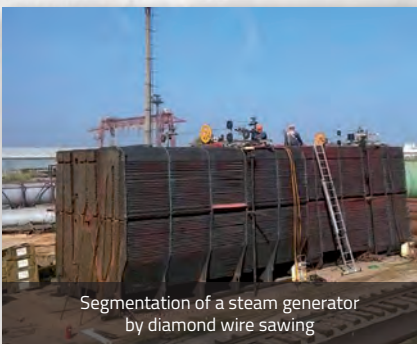
Plunge wire sawing of steel tubes in a nuclear power plant in Spain
